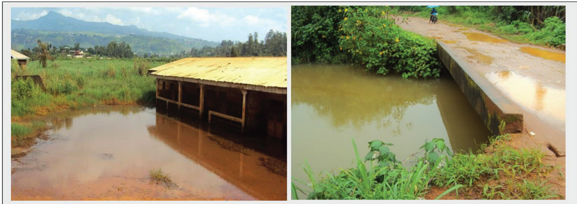
Figure 6 : Examples of flooding in Bamenda city (A = Mulang has abandoned house, B = bridge Ntamulung incorrectly calibrated).
