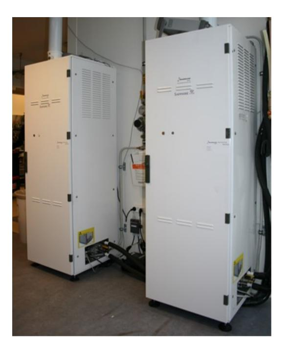
The SAPPHIRE consortium planned a test campaign on  $\mu$ CHP PEMFC systems, which was executed by partner Dantherm Power (today Ballard Power Systems Europe). The objective of the experimental campaign was to test two  $\mu$ CHP systems in nominal conditions for **3000 hours** of operation each, to provide a baseline for system degradation. Two stacks that had already been operated in a field trial for 5000 hours were selected to remove break-in effects.
