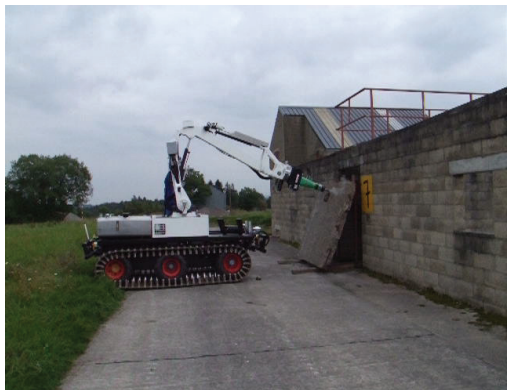
Figure 16. The LUGV uses its jackhammer to breach through a concrete plate (Source: ICARUS).
