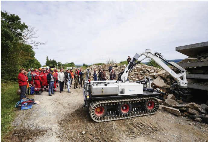
Figure 17. Debris clearance with the large UGV (source: ICARUS).
