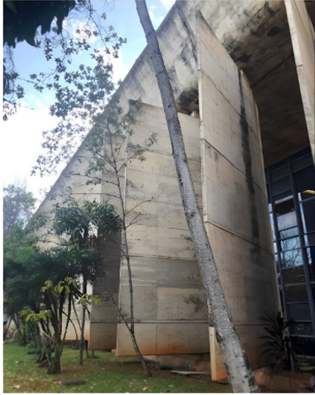
Figure 8 - Front facade. Source: Authors.
