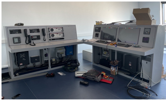
(a) The DNV/Bureau Veritas-compliant bridge during installation.
