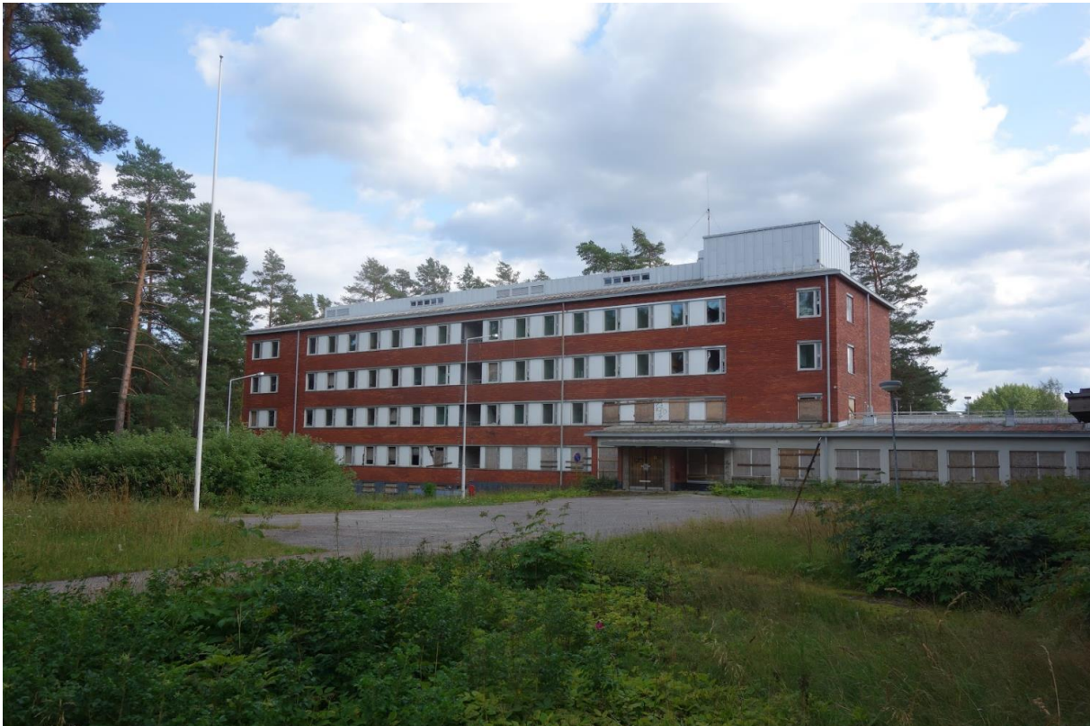
Figure 2. Demonstration building Tuukkala Hospital (Photo Esa Hannus)
