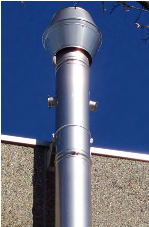
Figure 4-1 Examples of point sources. Vertical stack with free discharge (top left); vertical stack with rain-cap (top right); Y-shaped vertical stack with internal rain cap (bottom left); Horizontal stack (Bottom right). (Courtesy of Enviroware)
