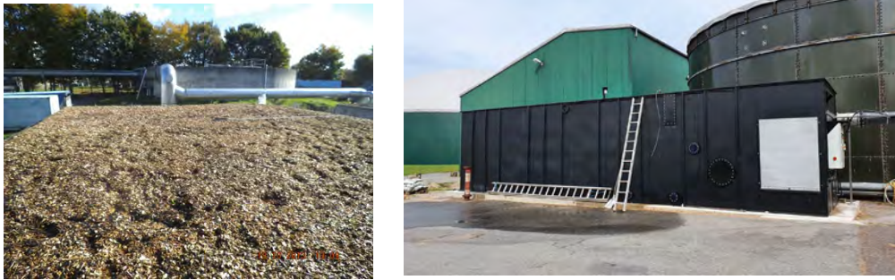
Figure 4-3 Example of active source: biofilter surface (left panel); biofilter container open on the top (right panel) (Courtesy of Olfasense)
