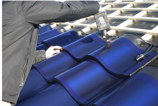
1.3. Crep s fotonaponskim sistemom (The Solé Power Tile, kompanije SRS Energy)
