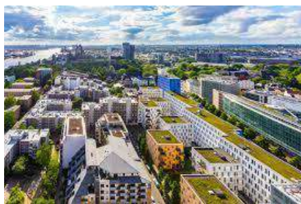
Figure 1 Green roofs in urban areas
