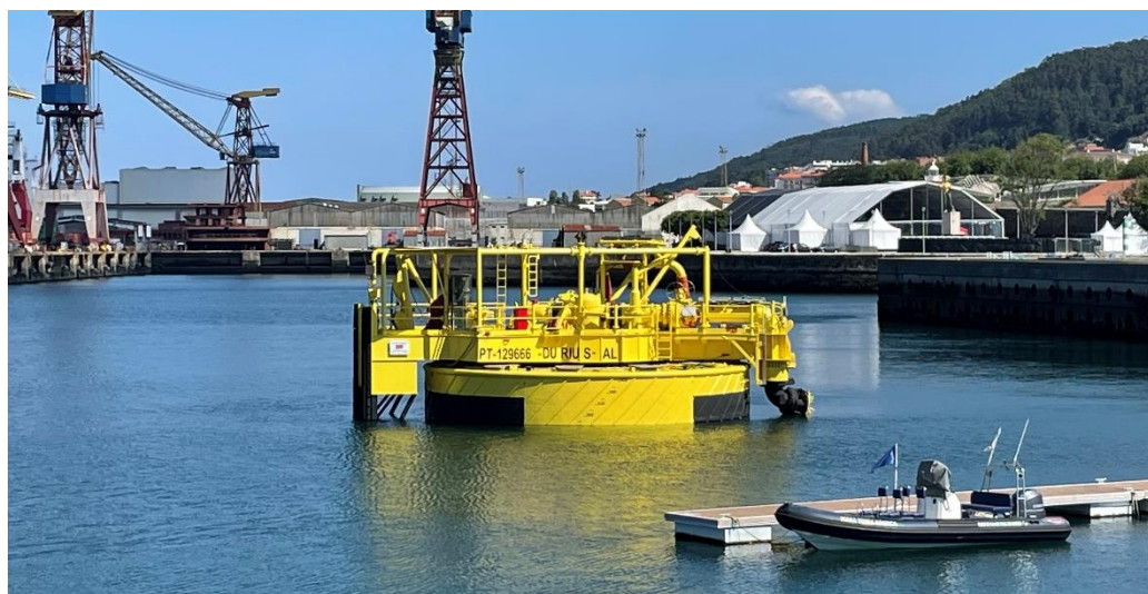
Figure 3-3 - Floating Structure installed on the Coastal Testbed of the ATLANTIS Test Centre
