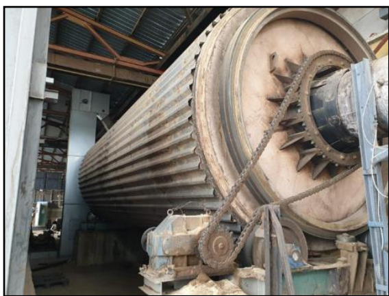
Fig.4. Tumble dryer (front) and chute (rear)
