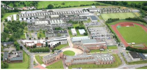
Fig. 3. Ariel view of the CIT Campus
