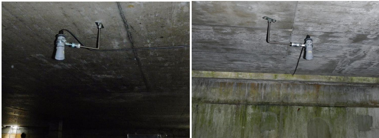
Figure 24: Ultrasonic water level sensors mounted in the reservoir s1: s1_h_us_maxbotix_1 (left) and s1_h_us_maxbotix_2 (right)
