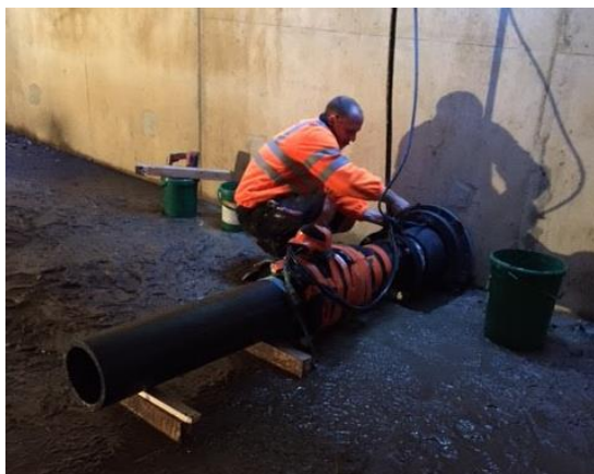
Figure 21: Installation of p1_q_mid_endress in the reservoir s1.
