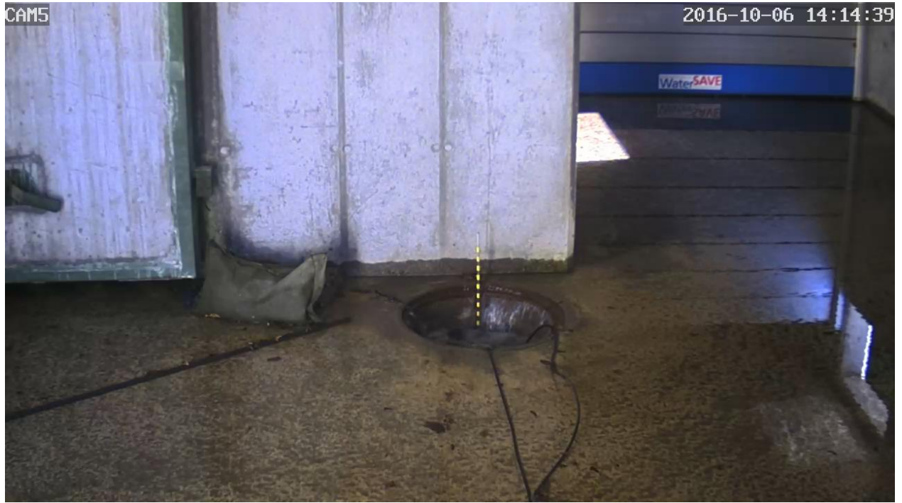
Figure 14: View from CAM5 of manhole m3, with ruler pole system emerging from hole.
