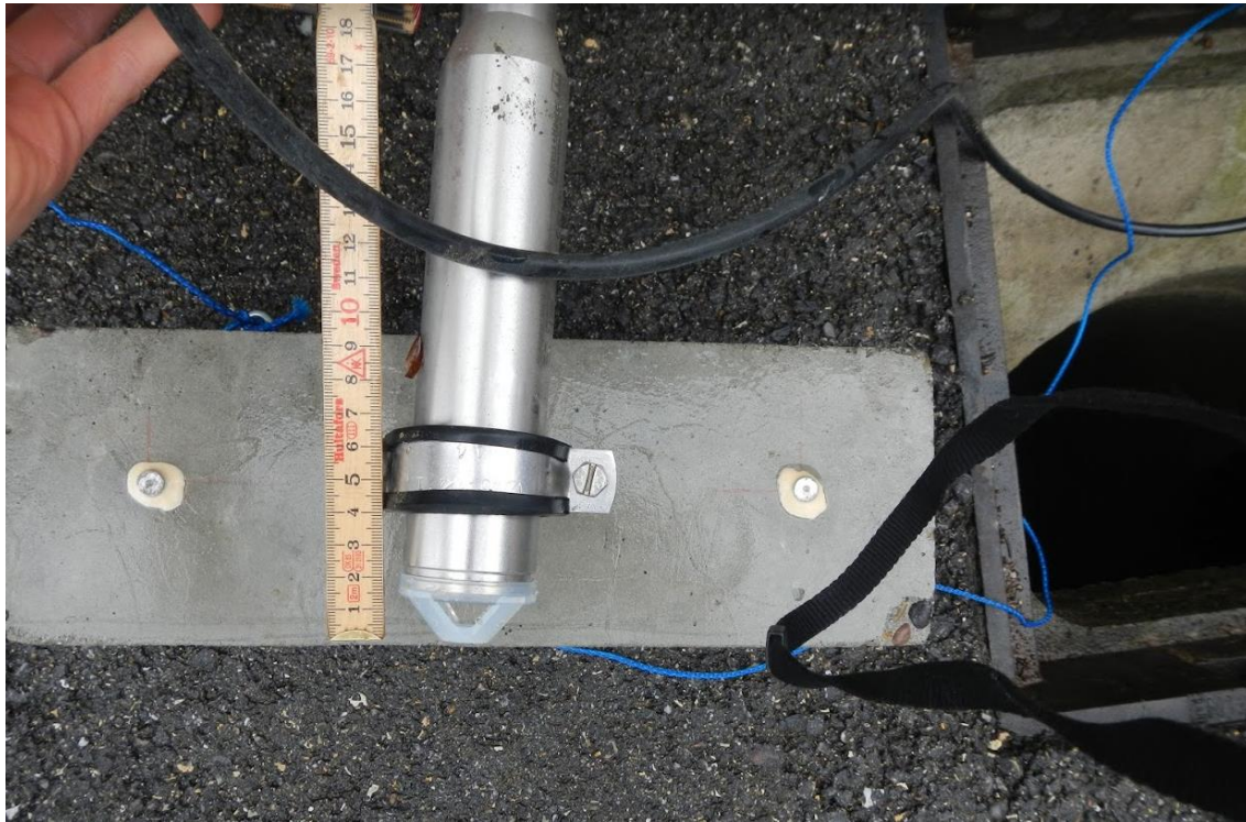
Figure 16: Sensor m1_h_p_endress that was placed in manhole m1.
