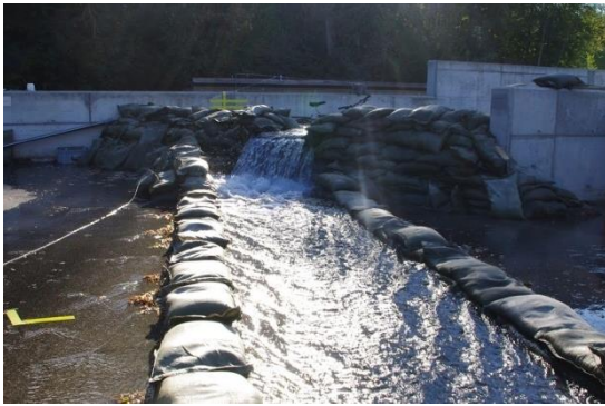
(a) Weir w1
