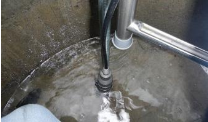
Figure 18: Installation of m2_h_p_endress in manhole m2.
