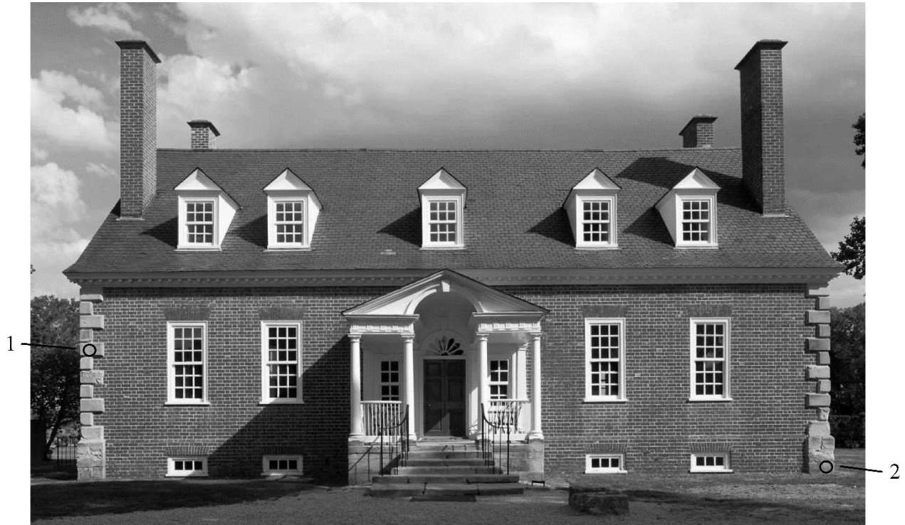
Figure 1 -- Picture of the north side of Gunston Hall, showing the location of the cornerstone sandstone blocks that contain a pterosaur wing impression (1) and foot impression (2). Image adapted from "Gunston Hall" by Stephen Brooke Studios (ca. 2012).
