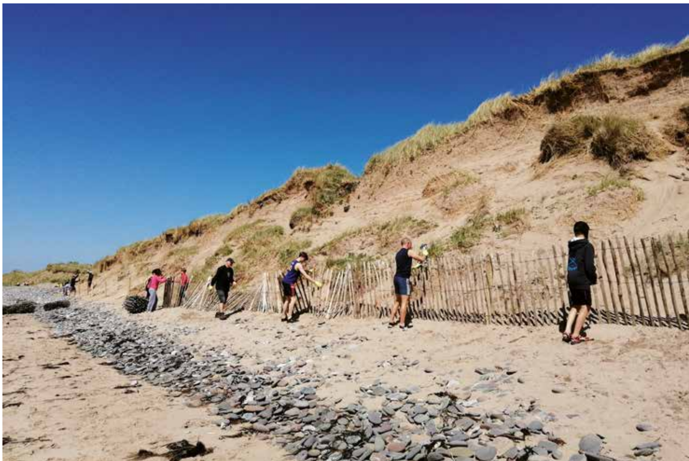
Figure 5.1 Example of community-led Nature-based Solution (installation of dune fences) to mitigate wind-blown sand leading to closure of the road in the Maharees Peninsula, Ireland.
