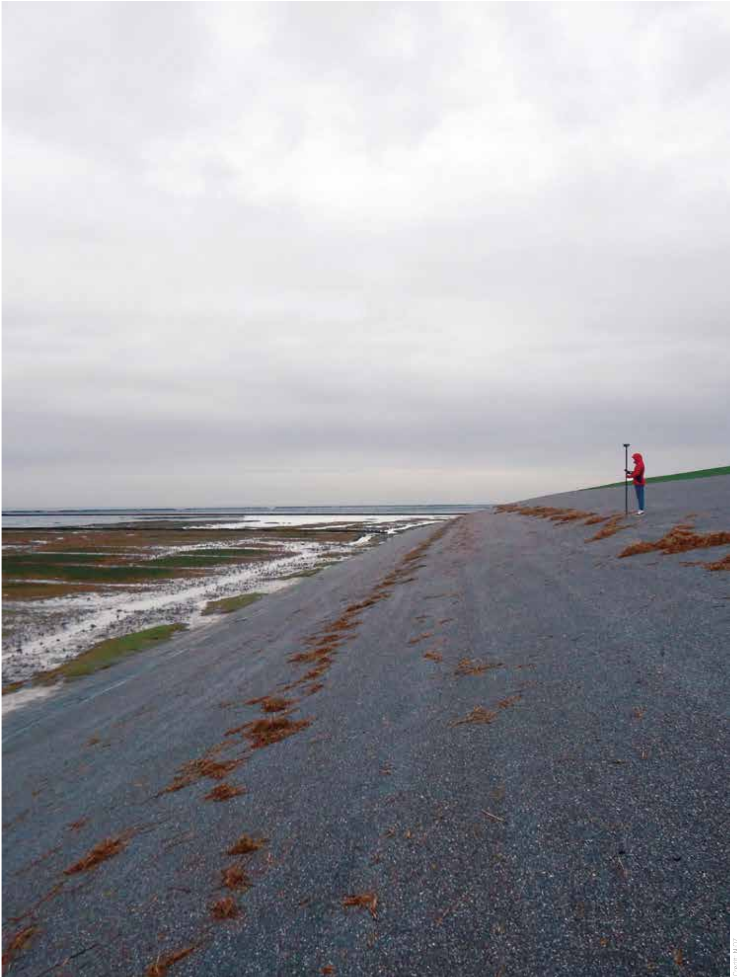
Measuring the position of flood marks on the dyke along the Dutch Wadden Sea.
