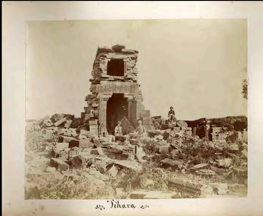
Sanchi. Temple 45 before clearance, showing seismic collapse
