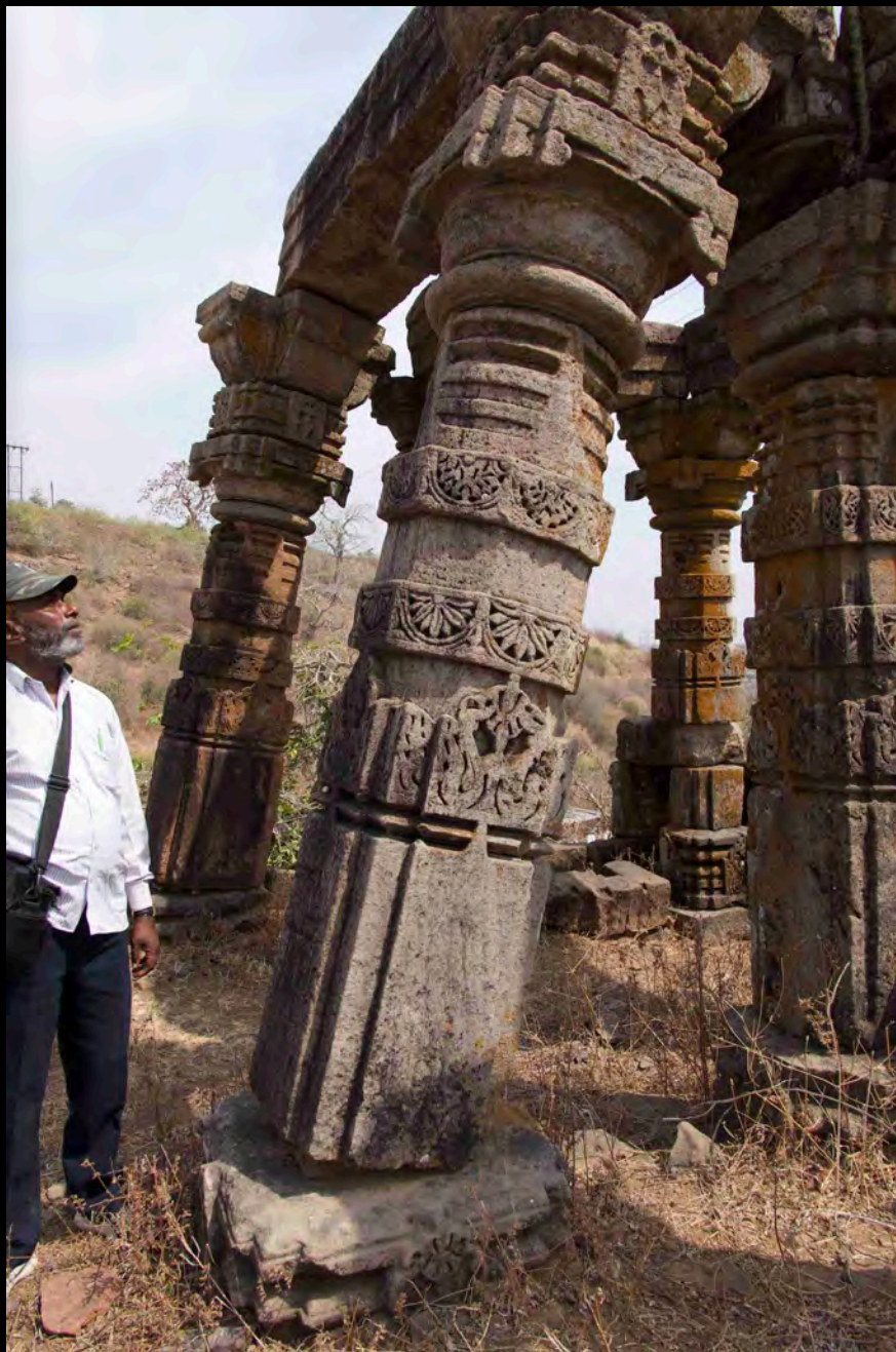
Omkareswar. Temple, about 1100, showing earthquake damage.
