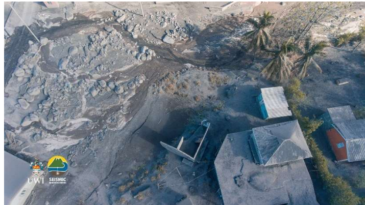
Figure 6.8 Lahar (mudflow) deposit, Sandy Bay Village. Jawid Collins, UWITV
