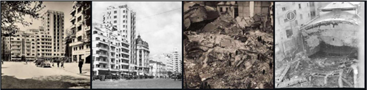
Figure 5.7 Carlton Building before and after the 1940 Vrancea earthquake (photo sources: muzeuldefotografie.ro/Cristian Laubach for the last image)
