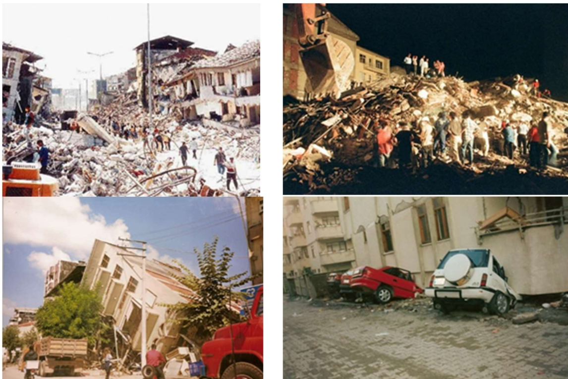
Figure 4.3a, 4.3b, 4.3c, 4.3d– Examples to building damage (Source: Sakarya Haber, access 2023)
