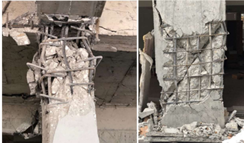
Figure 4.8 Collapsed mid-rise RC building
