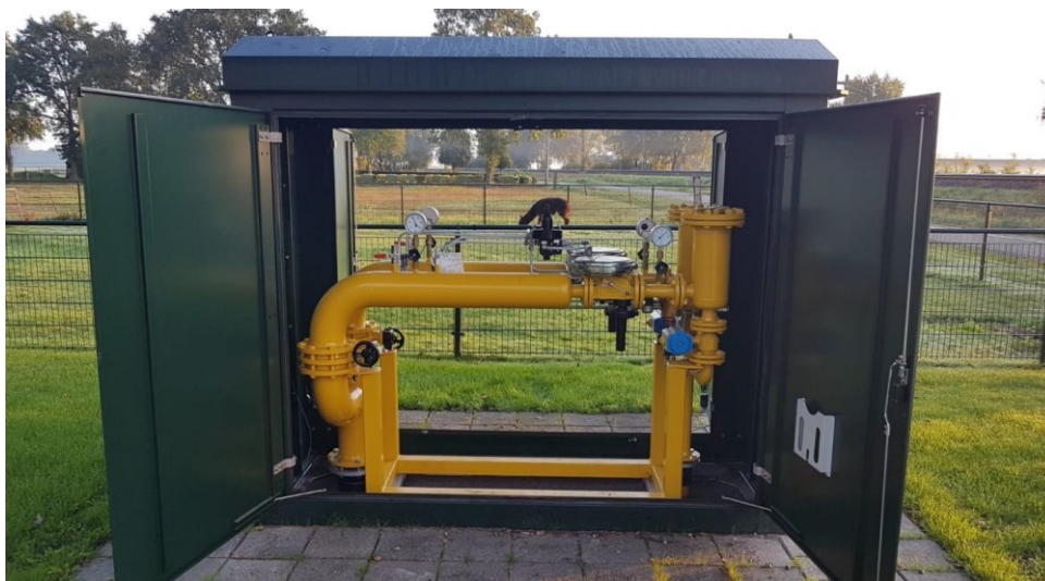
Figure 12 Concept of the gas pressure regulation station for the hydrogen-based district in Hoogeveen [20]
