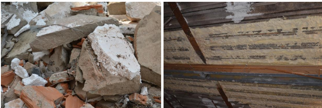
Figure 3. Examples of complex insulation materials that are difficult to dismantle (left: expanded polystyrene, right: polyurethane foam).
