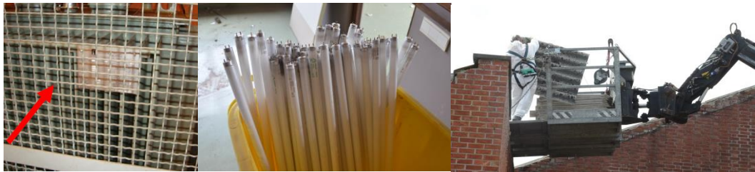
Figure 2. Hazardous materials (left: PCB-containing transformer, middle: mercury-containing lamps, right: asbestos).
