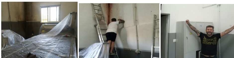
Figure 2: Our CNC mill after a fire in autumn 2020. It was recovered by associated, including professional painters.
