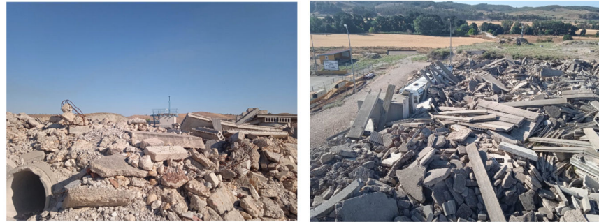
Figure 6. Images of the collapsed structures for the practice scenario.
