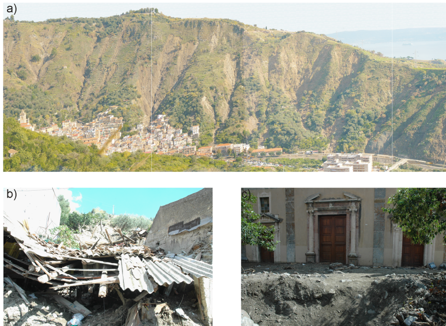
Figure 5: Photo-panorama of Giampileri village after the alluvial event: a) the slope scoured by debris flows; b) Giampileri urbanized area damaged by the alluvial event; c) Giampileri urbanized area where the sediment deposit level is recognizable.
