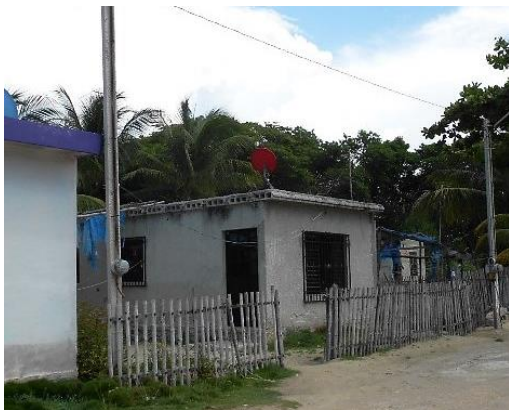
a) Typical substandard concrete masonry dwelling in Progreso (Yucatán, Mexico) (credit: F. Matta)
