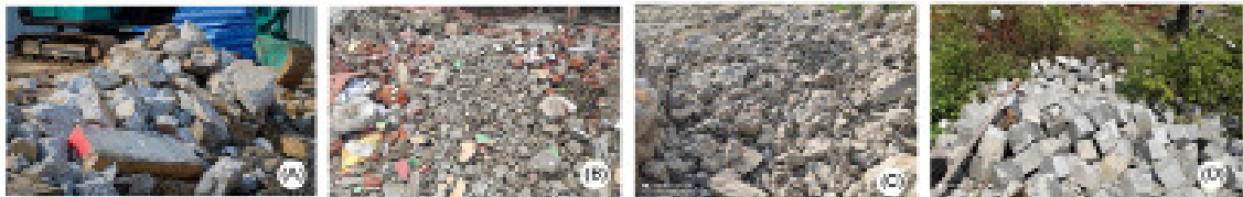
Figure 1: Construction and Demolition waste: (a) Demolished Concrete Waste at Bharatpur (b) Demolished Building Waste Bharatpur (c) Demolished Road Pavement at Gondryang-Pulchowk Road, Chitwan (d) Broken Concrete Cube Specimen at Laboratory
