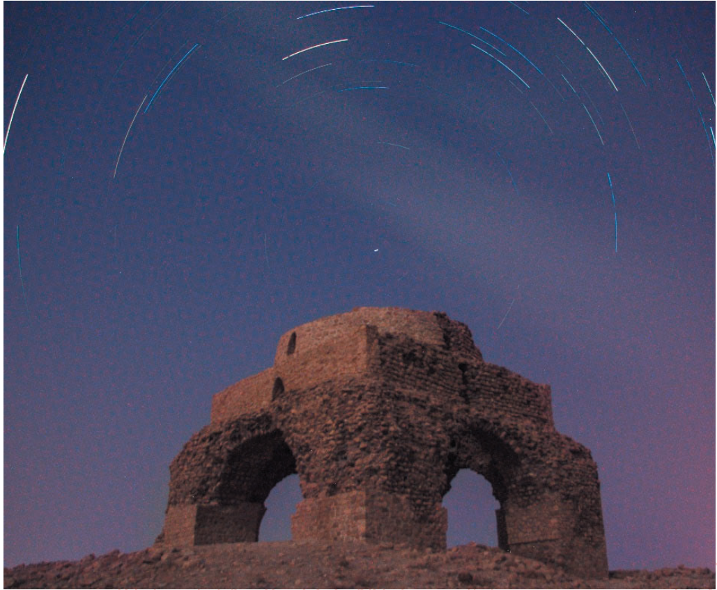
Fig. 26: The Chartaqui are very well oriented. They are structures consisting of four pillars oriented according to the cardinal points, and four arches that support a dome (Credit Hosein).
