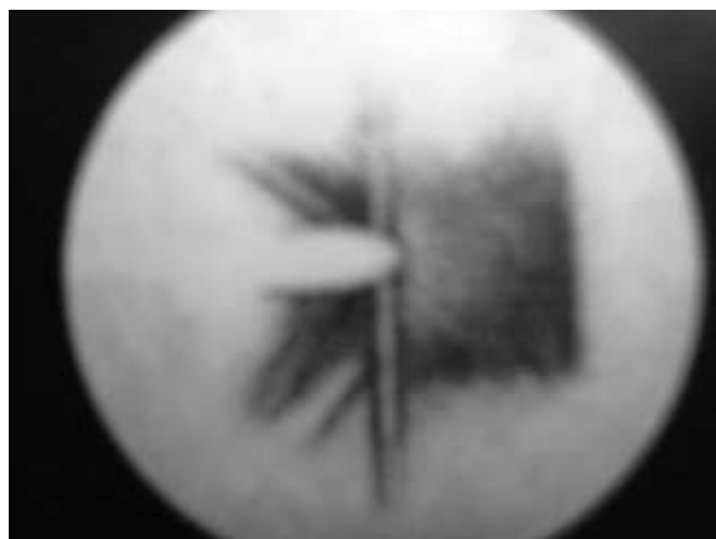
Figure 18-9: The last of the six photographs published by Mach and Salcher under the title Photographische Fixierung der Projectile und der Luft in the newsletter of the Viennese Academy in 1887.
