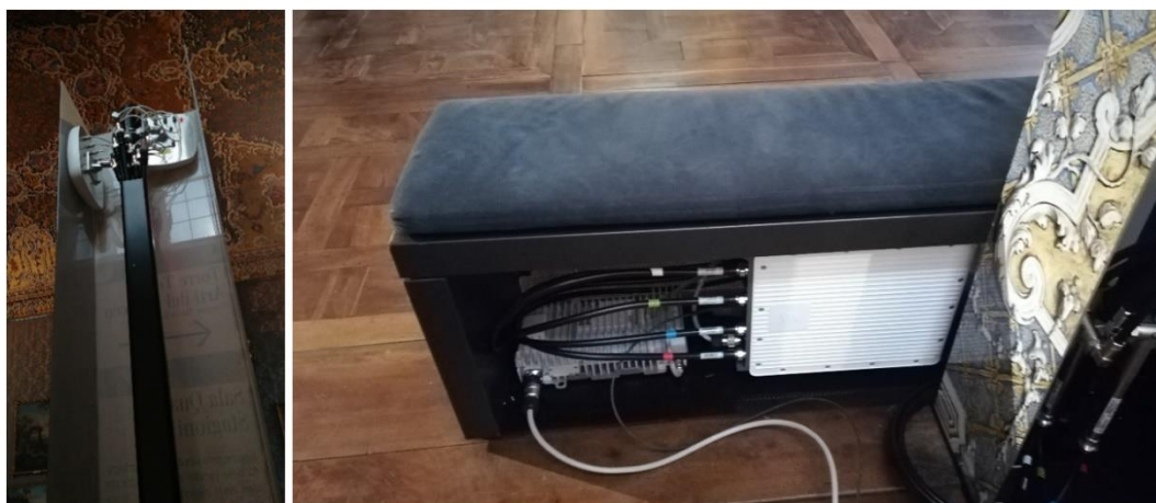
Figure 5. Installation detail and masking solution at Palazzo Madama.
