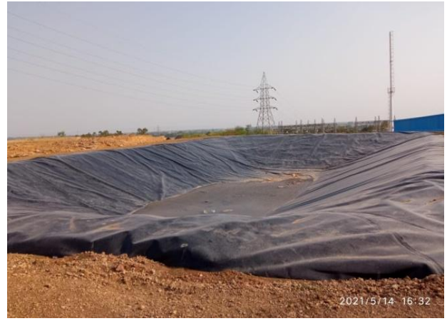
Sanitary Landfill Leachate collection pond
