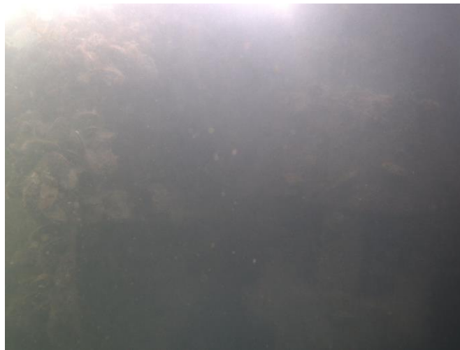
Figure 2-21: Visibility at less than one meter from the structure.
