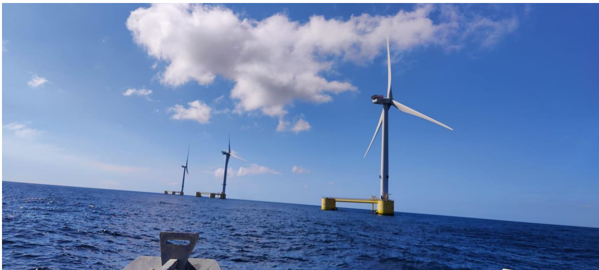
Figure 26: Offshore wind turbines photo taken from the boat.
