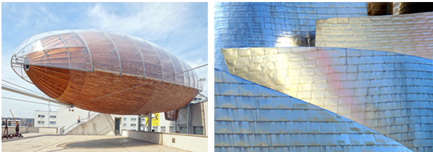
Figure 9.17 Example of parametric design: art installation titled Airship Gulliver (architect: Martin Rajniš, 2016). A galvanized steel structure was clad in timber in the form of a zeppelin and is externally protected by a layer of ETFE foil (left), and Guggenheim Bilbao Museum (architect Frank Gehry, 1991–1997; right).
