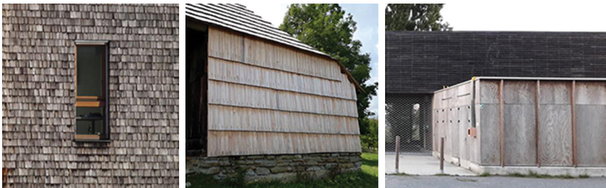
Figure 9.2 Plywood and wood shingles implemented on buildings.
