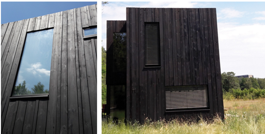
Figure 9.6 Building façade finished with Xyhlo biofinish technology. Courtesy of Michael Sailer, Xylotrade.
