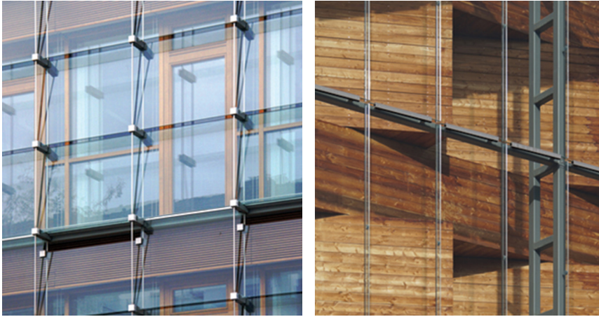
Figure 9.12 Example of ventilated envelope: (left) Hammer Strasse 19, Düsseldorf (architect: Petzinka Pink Architekten, 2000) and (right) Rheinisches Landesmuseum in Bonn (architect: Knut Lohrer, 2003).
