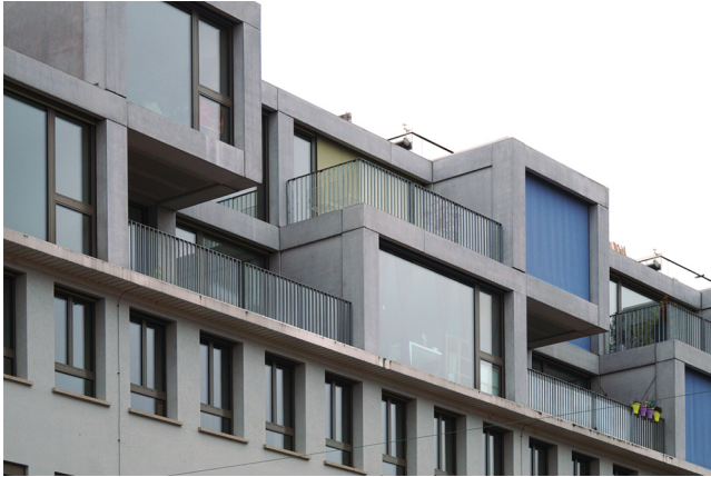
Figure 9.8 Implementation of timber for adding stories to existing buildings: Rauti-Huus (Spillmann Echsle Architekten, Zürich, 2015).
