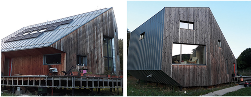
Figure 9.28 Passive wooden-straw family house in Melčice-Lieskové, Slovakia (Oximoron Studio M. Šichman, B. Meluš, 2013).
