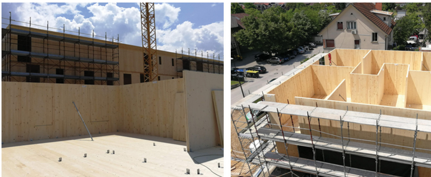
Figure 9.7 Construction process with CLT panels. Courtesy of CBD.
