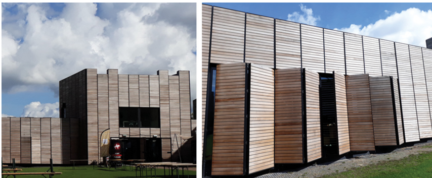
Figure 9.4 Façade from thermally modified wood: Castellum Hoge Woerd, De Meern, The Netherlands.
