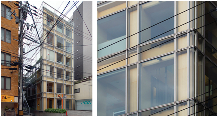
Figure 9.11 Example of a wood behind glazed curtain wall: the GC Osaka Building (architect: Shigeru Ban, 2000).
