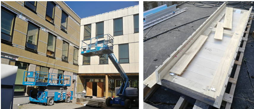
Figure 9.18 Prefabricated timber façade elements allowing a fast construction process.
