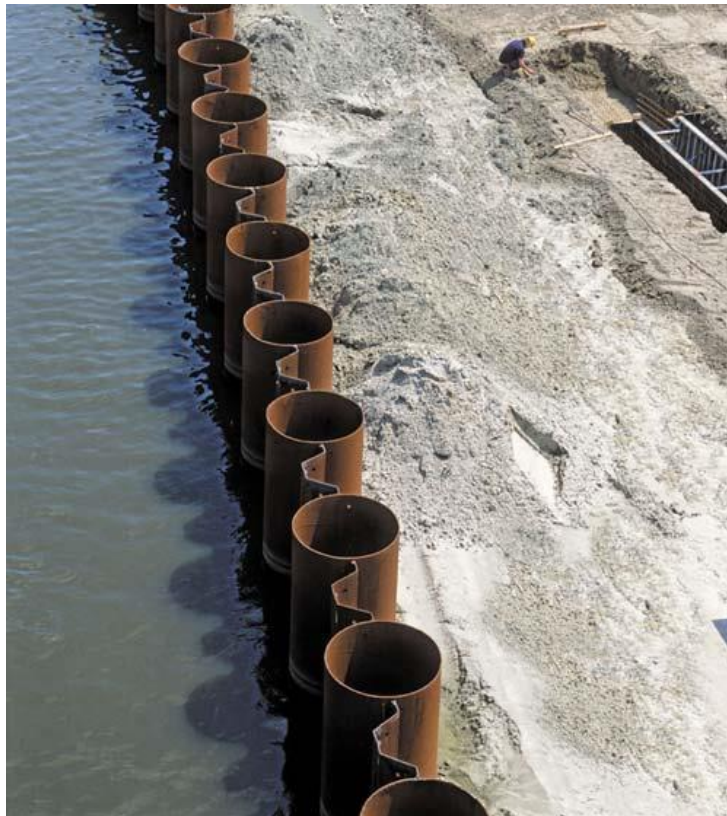
Figure 14 Typical Combi Wall Construction ( https://constructalia.arcelormittal.com/en/products/combined_walls )
