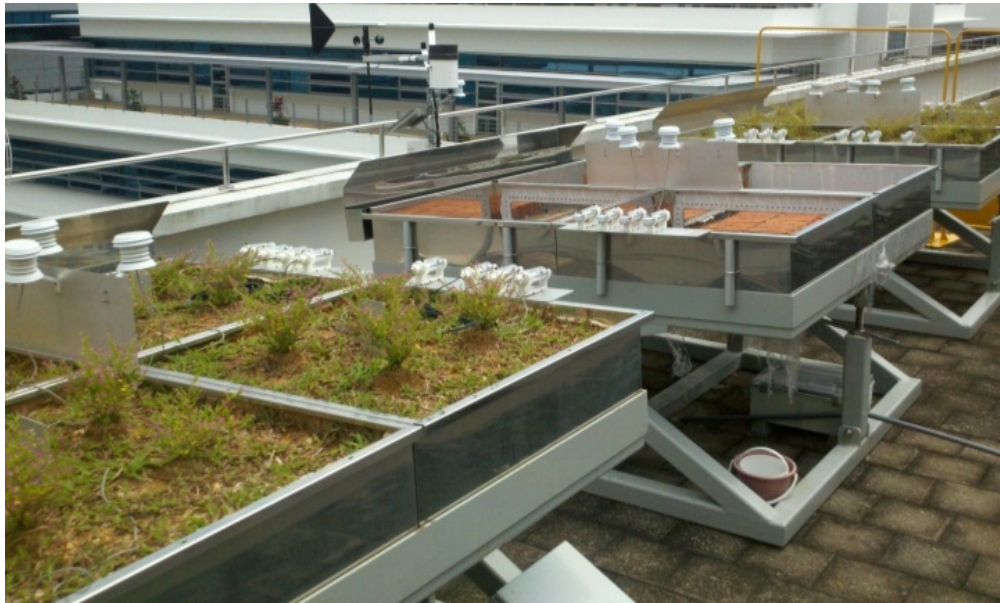
Fig. 1. Green roof test bed on the roof of academic complex N1 in NTU Three units of planter boxes are deployed; the middle one is the bare roof control.
