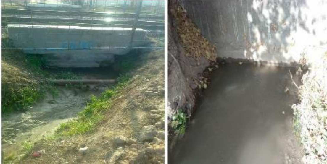
Figure-3. Condition of culverts in the first quarter
