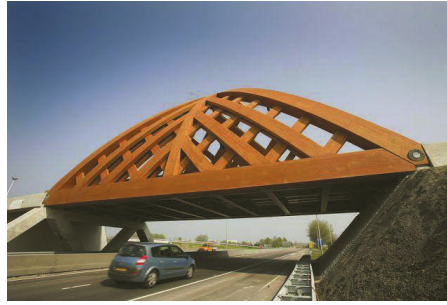
Figure 1.68 Sneek bridge in The Netherlands, constructed using Accoya™.
