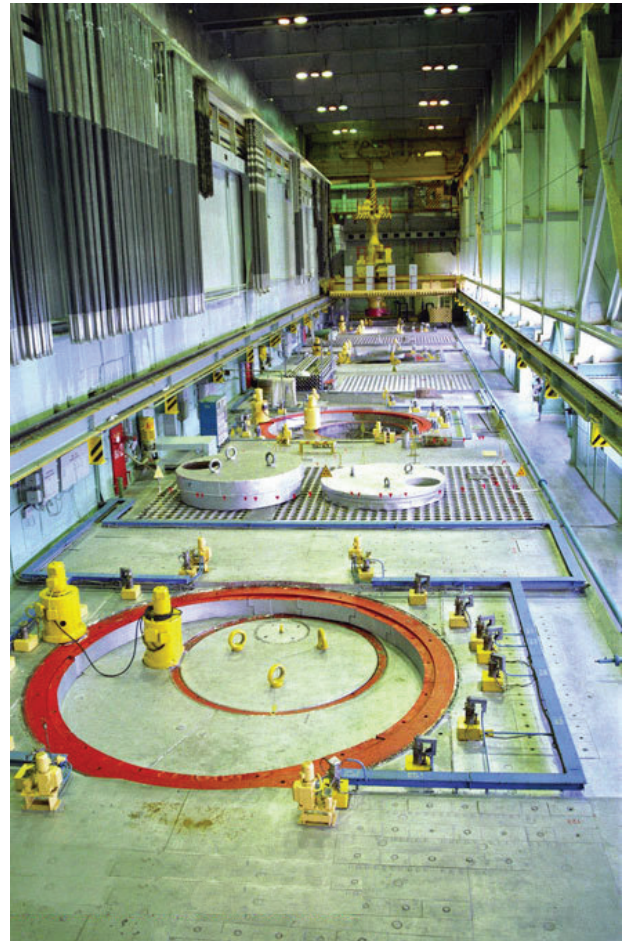
Figure 1. Bilibino NPP's central hall with four EGP-6 reactors [www.fotoalbum.su].
