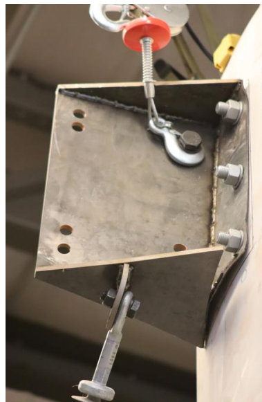
c) UC welding fracture under loading
