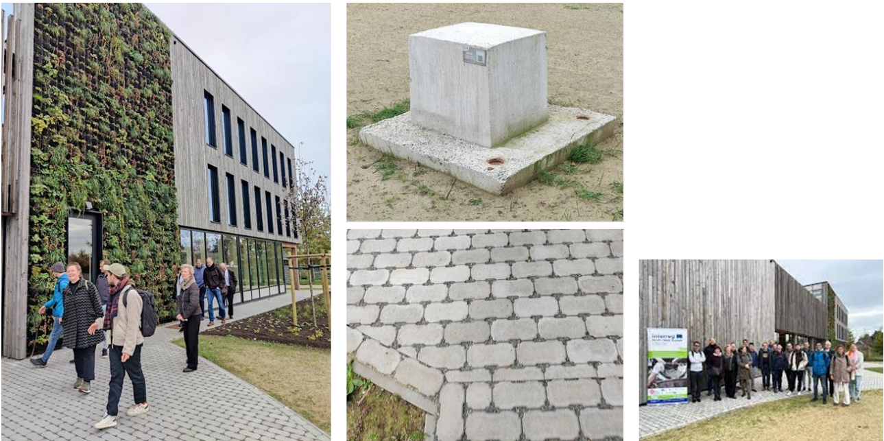
Figure 9-22 Circular office building in use with AAM pavers and with AAM foundation elements (extra element put next to the building for show-casing purposes)
