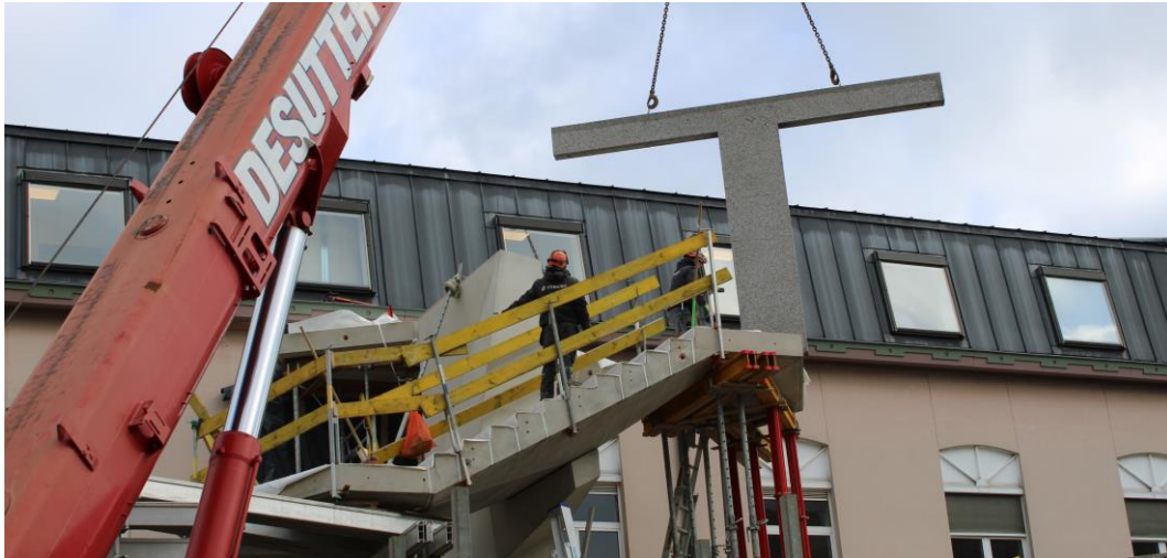
Figure 9-19 Installation of the T-frame at the school
