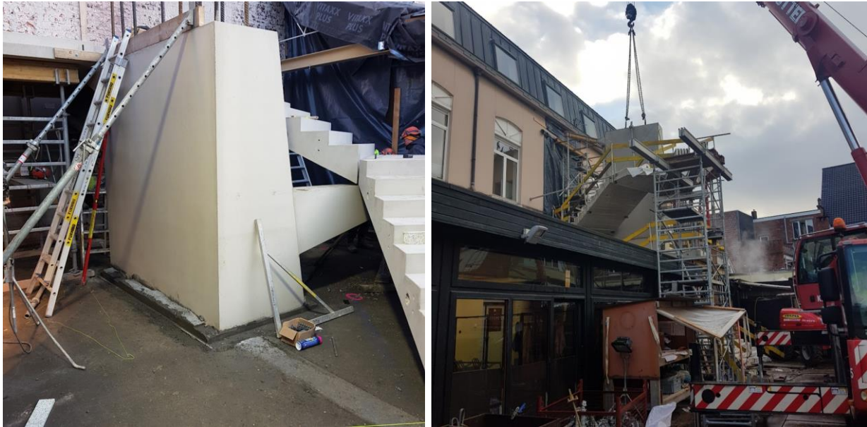
Figure 9-18 Installation of the precast members at the school
