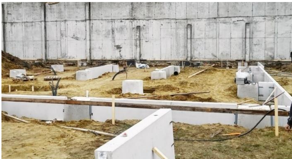
Figure 9-21 Installation of precast foundation elements (picture back end shows existing building)
