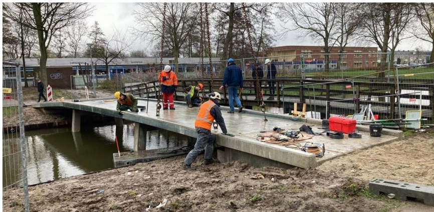
Figure 9-10 Lifting the decks in place
