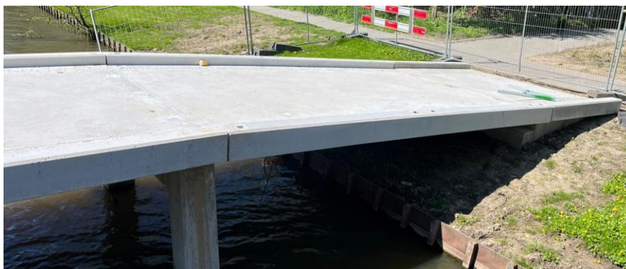
Figure 9-11 Final decks, awaiting gravel layer and railings
