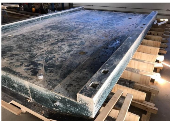
Figure 9-9 Side span after demoulding still showing dark green-blue colour
