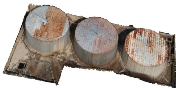
Fig. 2: 3D Model of the Inspected Site
