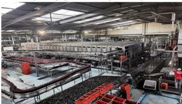
Fig. 2. Overview Image of The Equipment
