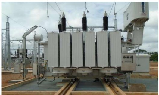
Figure 2:- 90/16.5 kV transformer; 40 MVA installed in Vridi.
