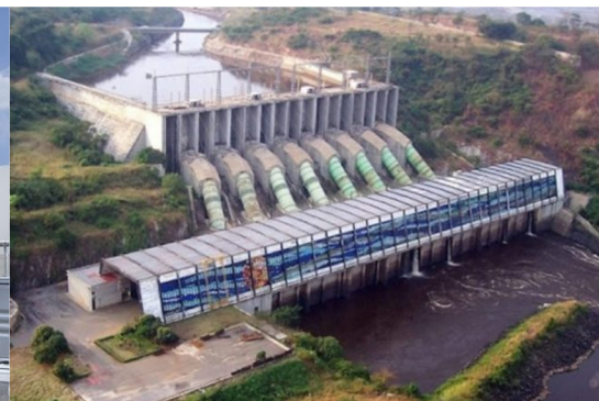
Nachtigal Dam Source : World Bank, Cameroon
