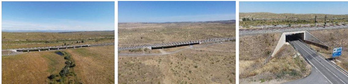
Figure 13 Railway bridges on the line Madrid-Bajadoz
