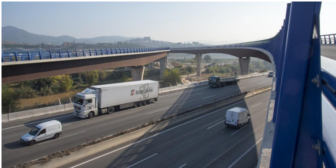
Figure 14 PR-04-B015 bridge (Łukaszewska, A., 2021)
