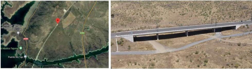
Figure 10 Location and overview of La Plata Viaduct
