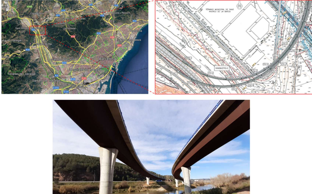
Figure 21. Location and general view of PR-04-B015 bridge
