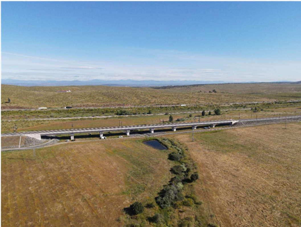
Figure 43. Valdelinares Viaduct. Drone view
