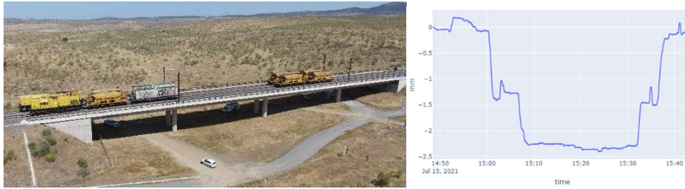
Figure 12 Load test of La Plata bridge and a sample of collected sensor data
