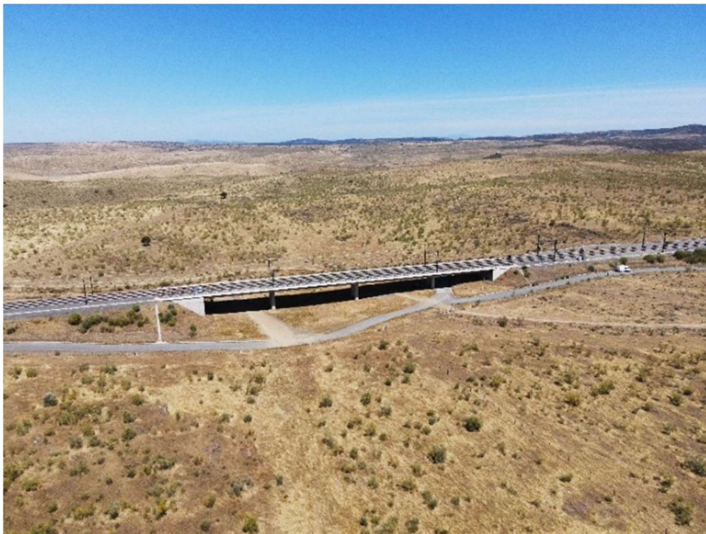
Figure 45. La Plata Viaduct. Drone view
