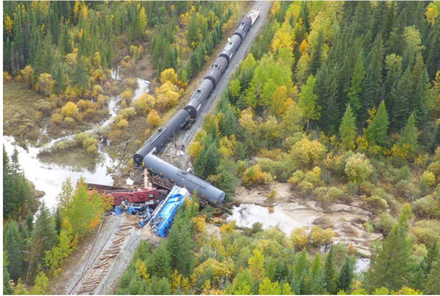
Fig. 9. Derailment on the Hudson Bay Railway line associated with flooding in 2018 Photo credit: Transport Safety Board of Canada, investigation R18W0237 (by permission).
