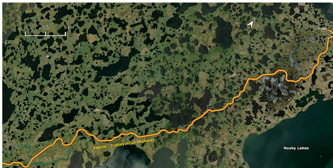
Fig. 6. The Inuvik–Tuktoyaktuk Highway (ITH) in Canada’s Northwest Territories. This illustrative section of the highway shows the engineering challenges for routing across the landscape while protecting the abundant freshwater resources, including the Inuit subsistence fishery in Husky Lakes. Source data: CanVec, NRCan (Open Government Licence—Canada), and ESRI High-Resolution Imagery (ESRI, Maxar, GeoEye, Earthstar Geographics, CNES/Airbus DS, USDA, USGS, AeroGRID, IGN, and the GIS User Community). Rendered with QGIS v3.14 (GNU General Public License).
