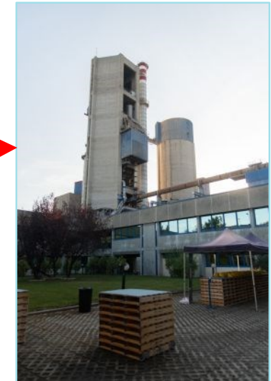
CO 2 capture pilot cement plant opened in October 2020 at Vernasca Cement plant
