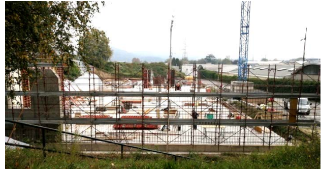
Figure 2. Construction site as of 19/10/2021.
