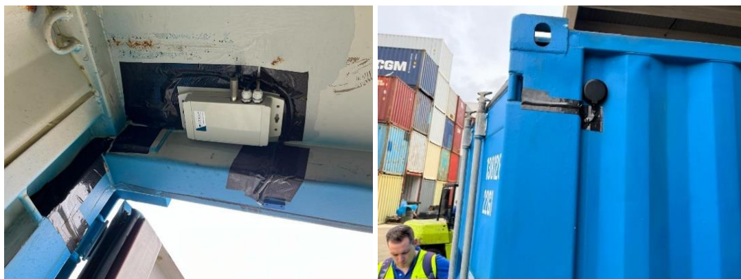
Figure 49: Final demo device installation
