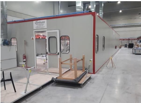
Figure 8 Sanding area cabin (exterior)
