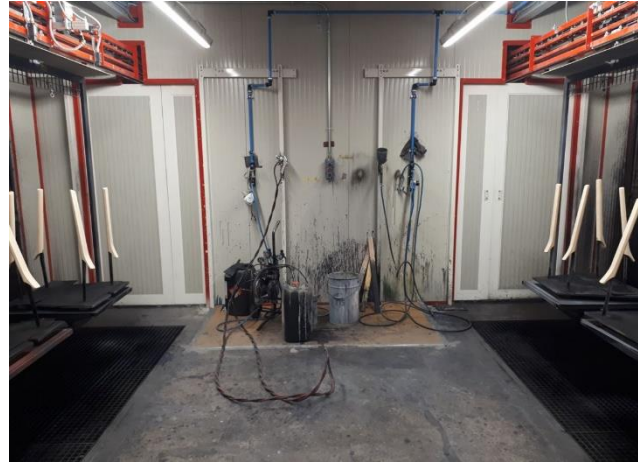
Figure 5 Staining area cabin (interior)
