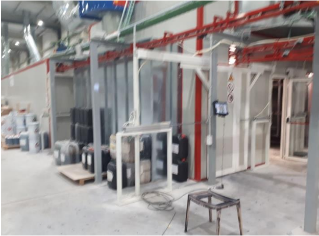
Figure 4 Staining area cabin (exterior)
