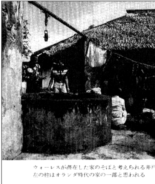
Santiong House and well, 1980. “The well that is beside the house where Wallace was thought to have lived; I think the cement column is from Dutch times”. (Niizuma, 1997, p. 230)
